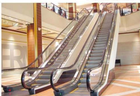
Atlantic Terminal New York, USA
