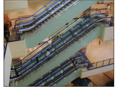
Light Under Handrail
